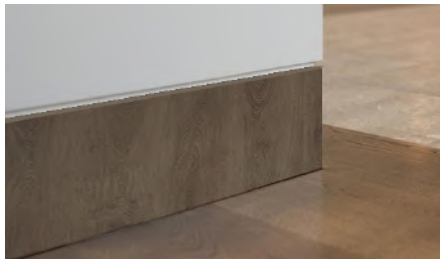
BASEBOARD - STAINED WOOD Finish to Match Millwork
